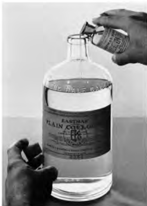
IODIZING THE COLLODION
