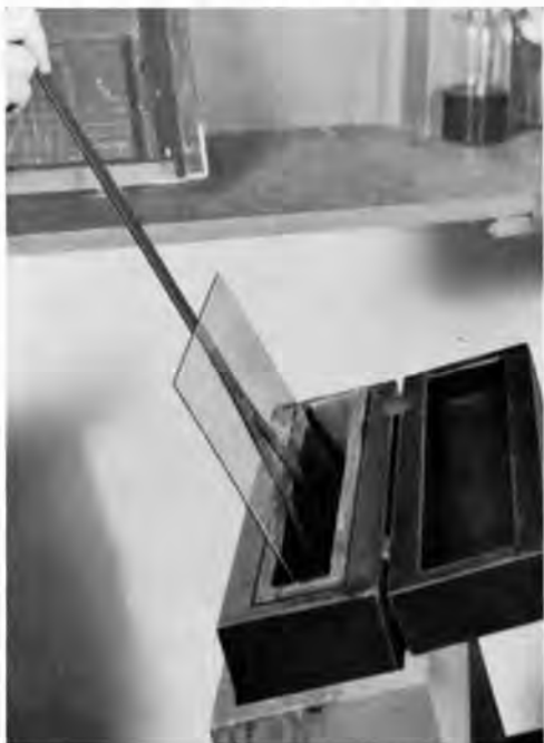
DIPPING THE COLLODIONIZED PLATE INTO THE SILVER BATH
